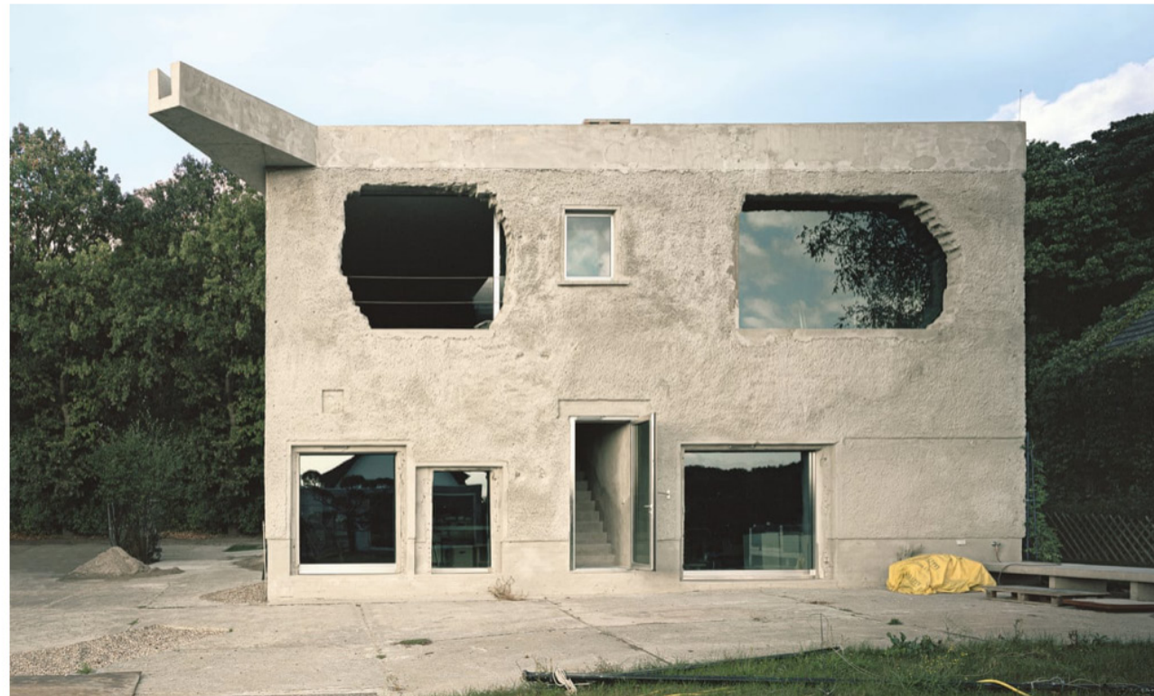
Build back better ... Arno Brandhuber's Antivilla in Krampnitz, Germany. Photograph: bplus.xyz
